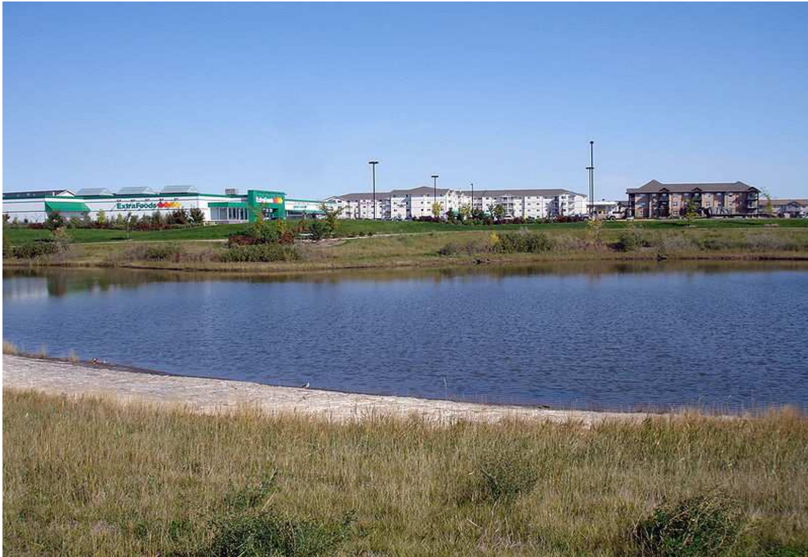
Retention basin for controlling urban runoff
