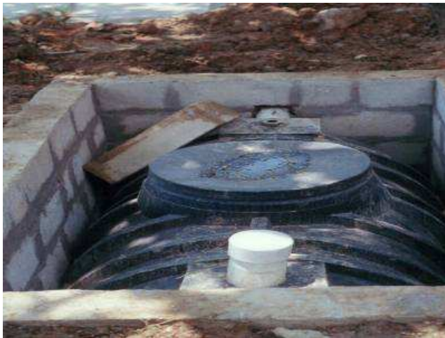
The septic tank partially installed in the ground
