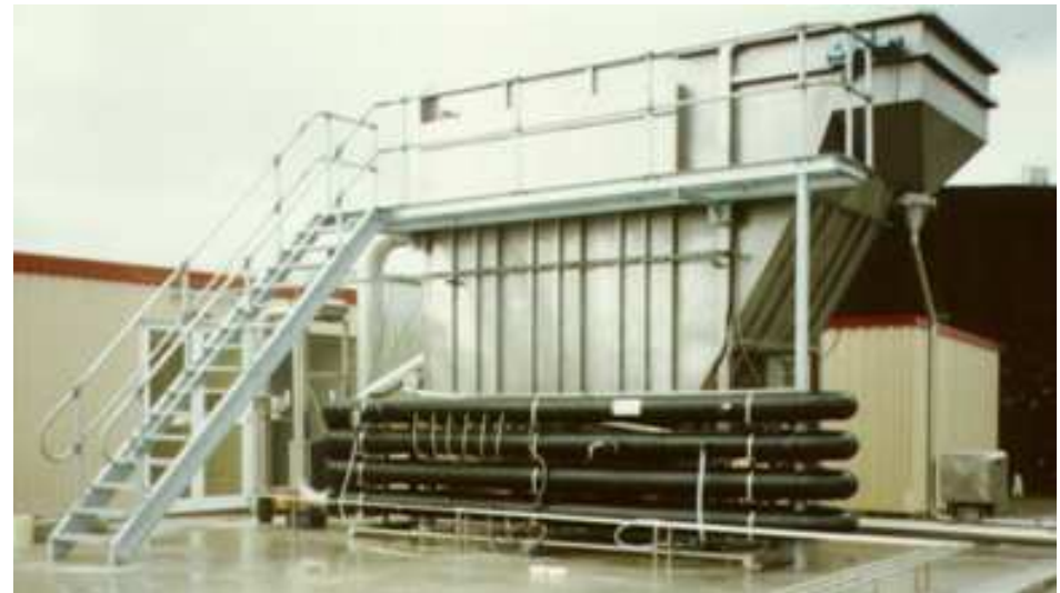
Dissolved air flotation system for treating industrial wastewater
